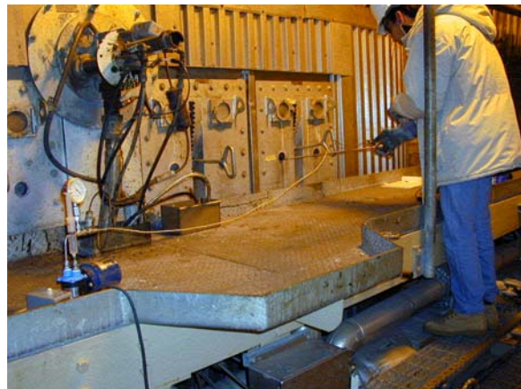
Figure 1. In-situ monitoring of high-corrosion areas.
